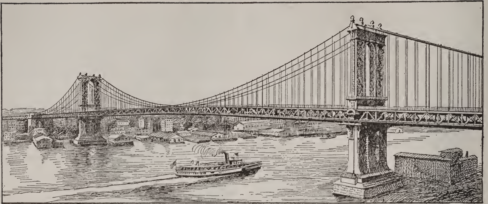
MANHATTAN BRIDGE, NEW YORK CITY
